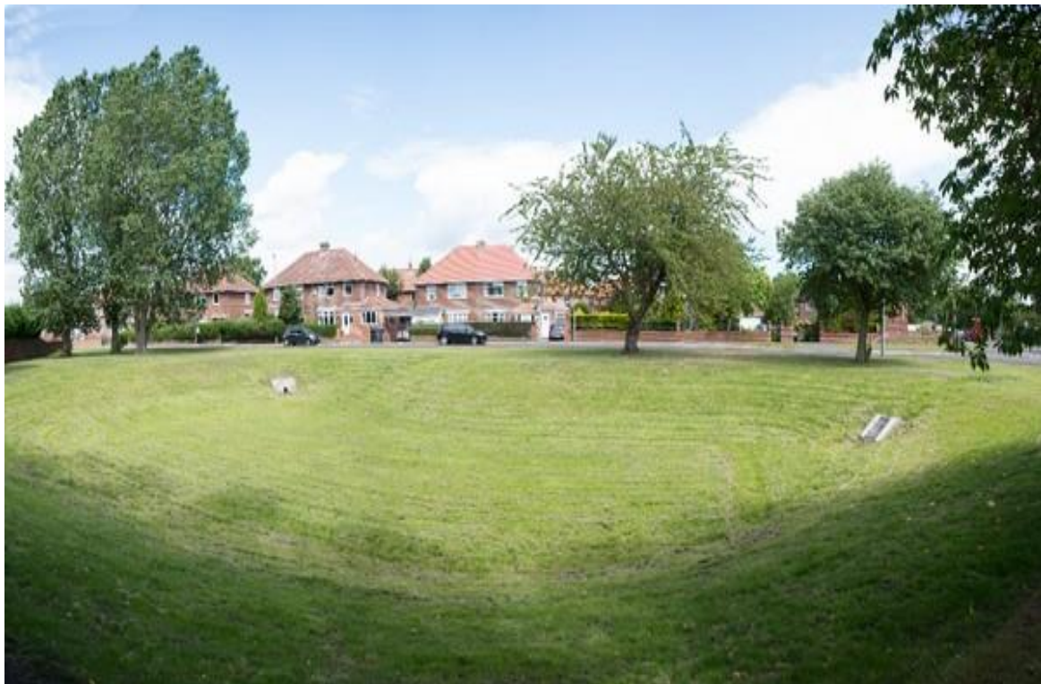
Figure 2 Completed detention basin
