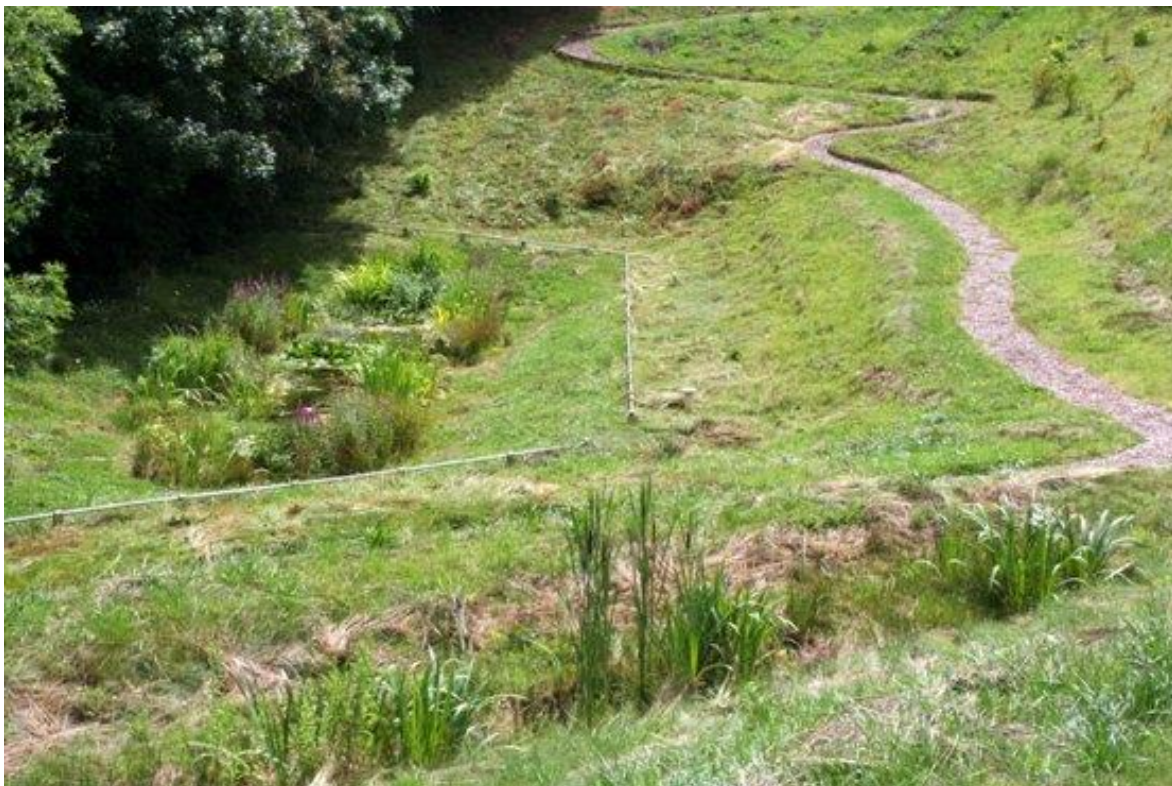
Figure 4 Low-flow channel to pond and outfall (Bob Bray)
