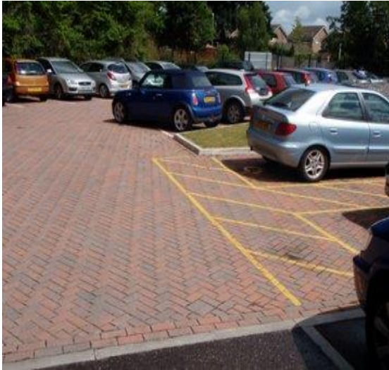
Figure 2 Permeable paving in school car park (Bob Bray)
