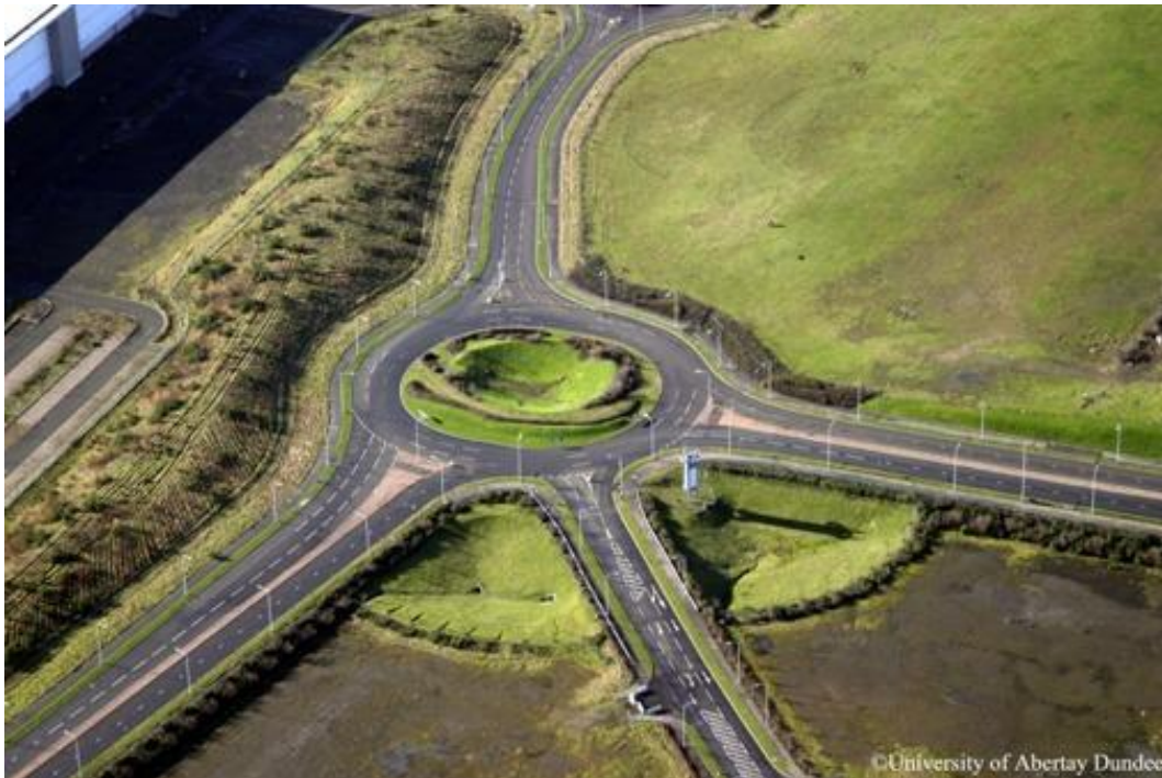
Figure 1 Detention basin DEX Roundabout
