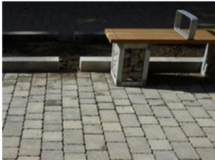
Figure 7 Permeable block paving
