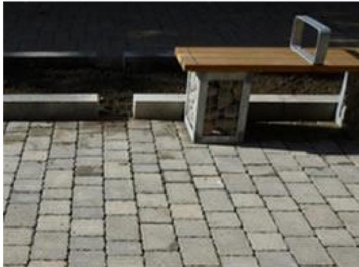
Figure 7 Permeable block paving
