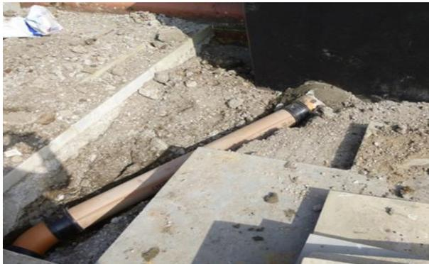
Figure 11 Connecting the overflow chamber of the attenuating planters to the rain garden via a clay pipe
