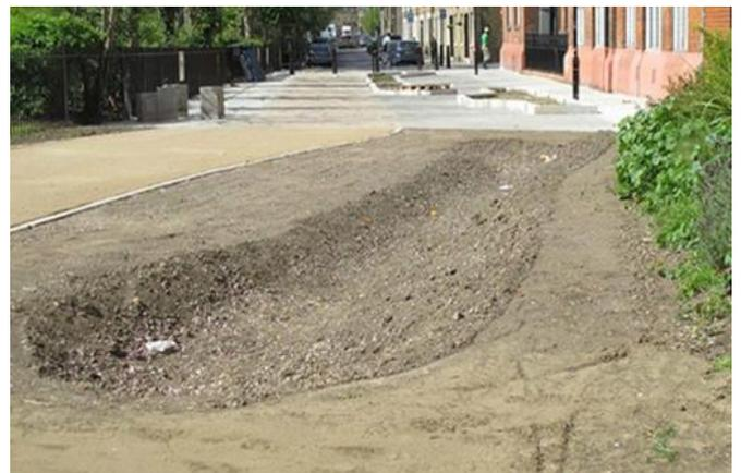
Figure 13 The swale formed
