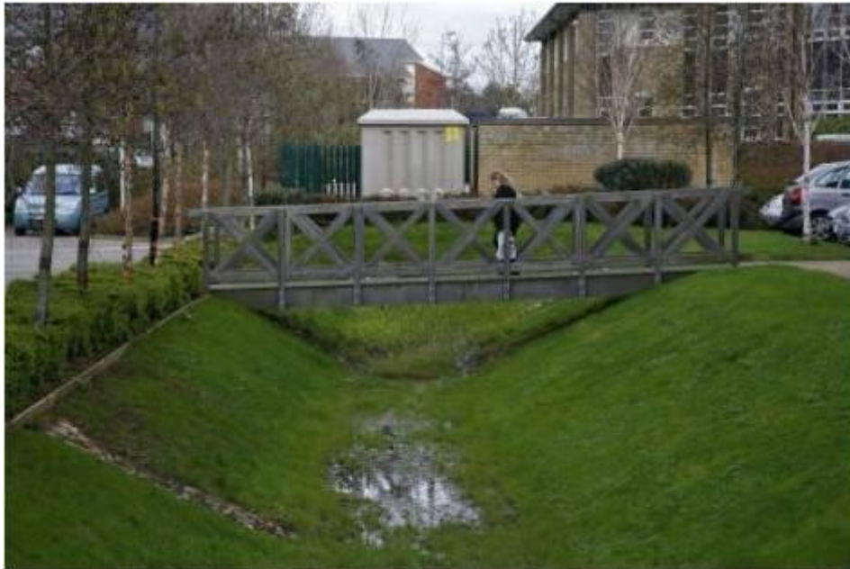
Figure 2 Swales, which take water from the paving, create attractive features in the business park (CABE/Stephen McLaren)
