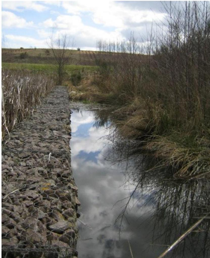
Figure 3 Stilling pool and gabion in system 2 reed bed 2
