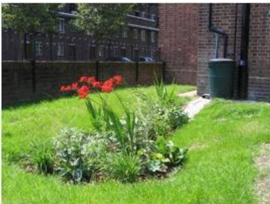
Figure 3 The rain garden once it had been constructed
