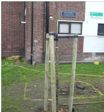
Figure 5 Image showing the recently planted tree and the rain garden redesigned around the underground services
