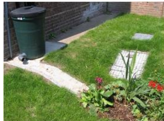
Figure 4 Water from the water butt flows into the rain garden
