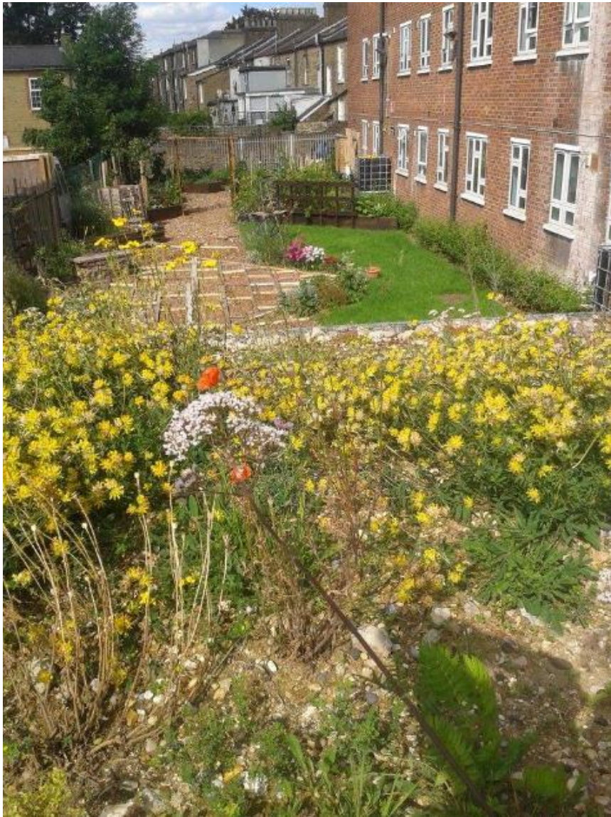
Fig 4: View of site from green roof with decking area under construction
