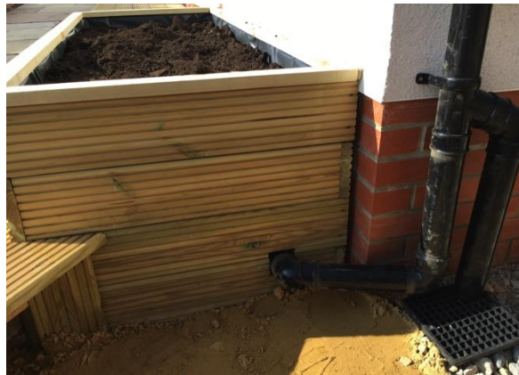
Downpipe connection to raised bed & overflow
