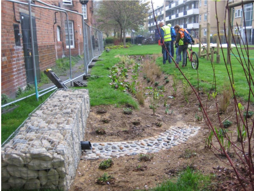
Rain Garden during construction
