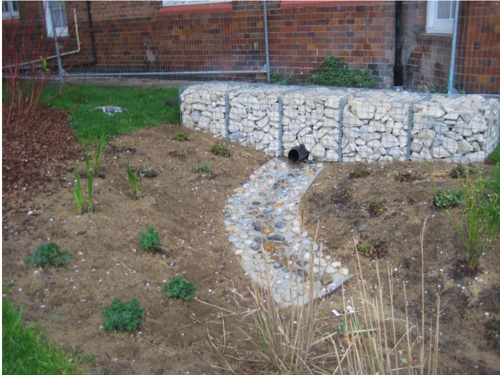
Gabion Header Wall and discharge pipe at completion
