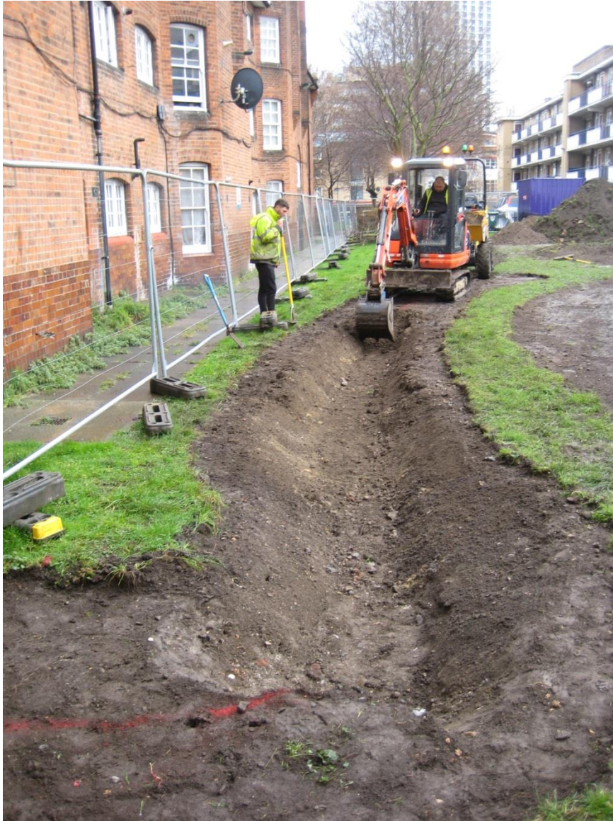
Rain Garden Progress – site excavation
