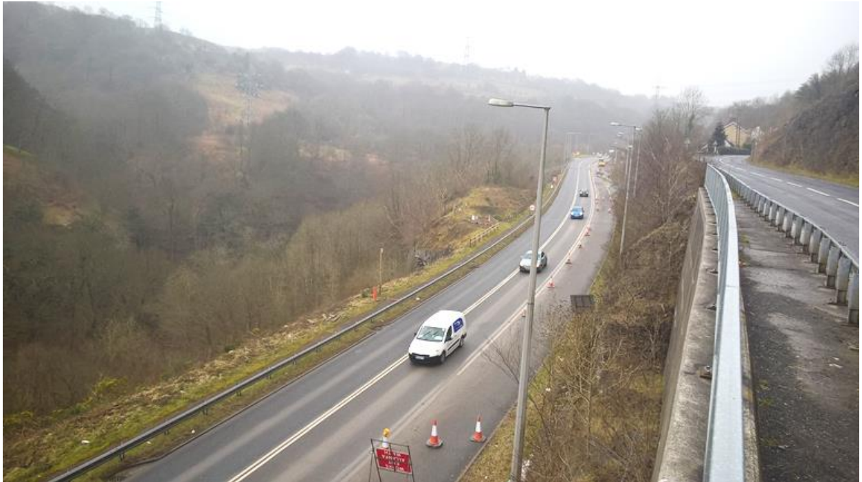
Fig 2: Existing road showing difficulties in terrain / topography
