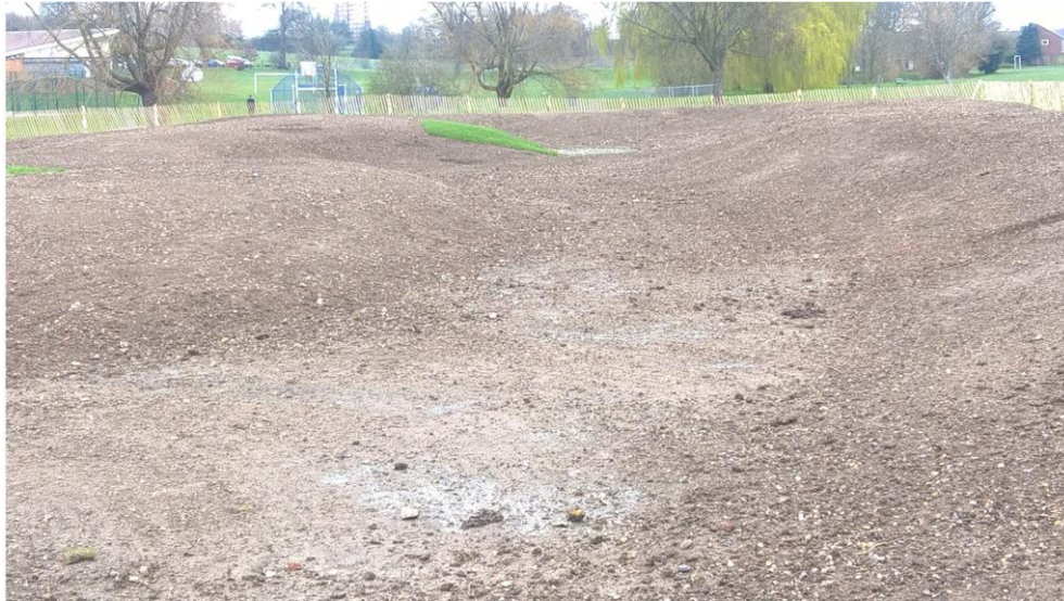
Figure 2: Swale during construction phase – unseeded
