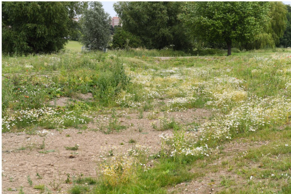
Figure 3: Swale further to establishment of vegetation July 2019
