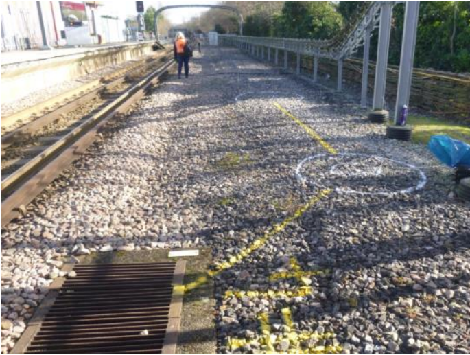
Fig 2: Setting out works
