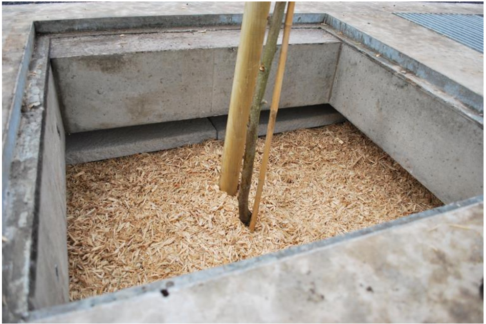
Fig 3: Installation of mulch layer
