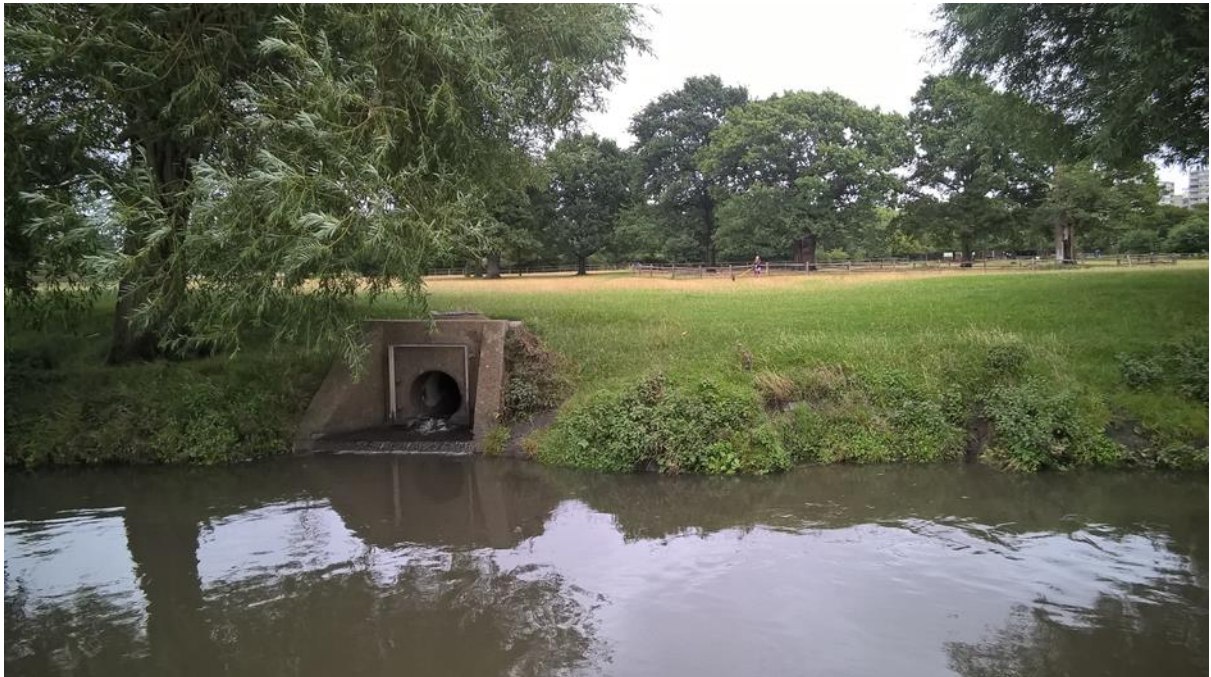
Fig 3: Existing Outfall to Beverley Brook
