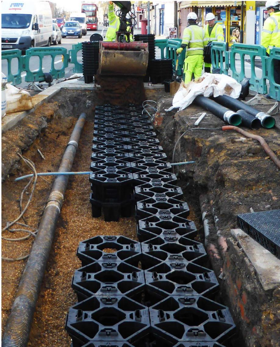
Fig 3: Tree pit cells being filled during construction
