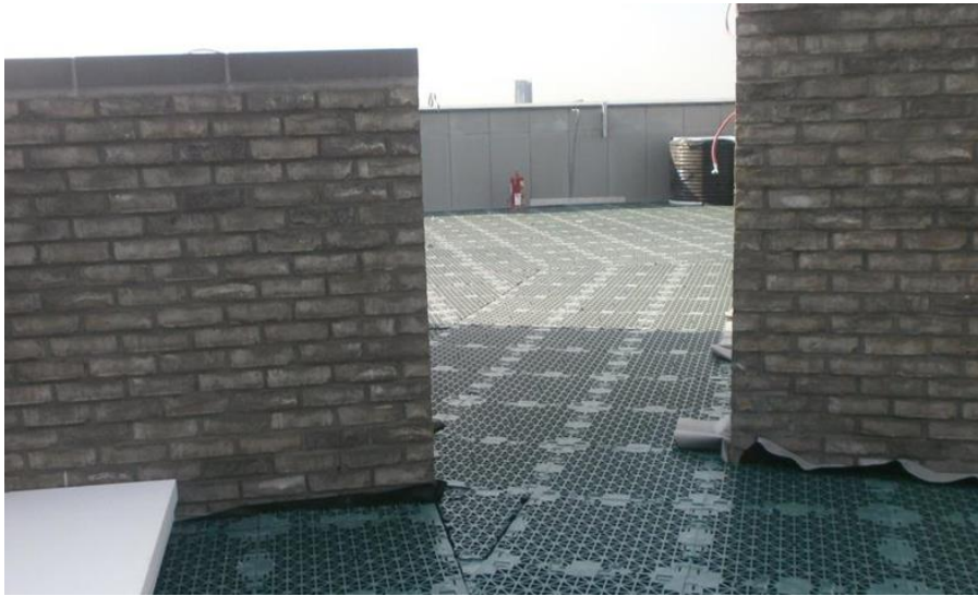
Fig. 3: Installed Void formers fitted in tight working environments
