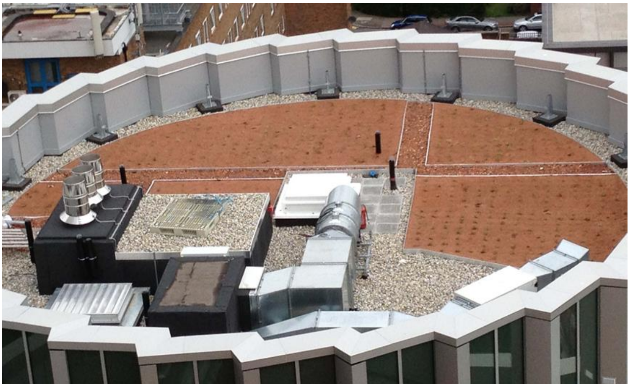
Fig. 8: Mixed finish roof
