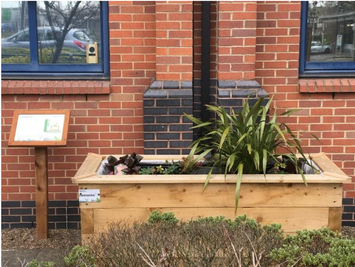
Figure 1 Rainwater garden at NWG's Boldon House, County Durham
