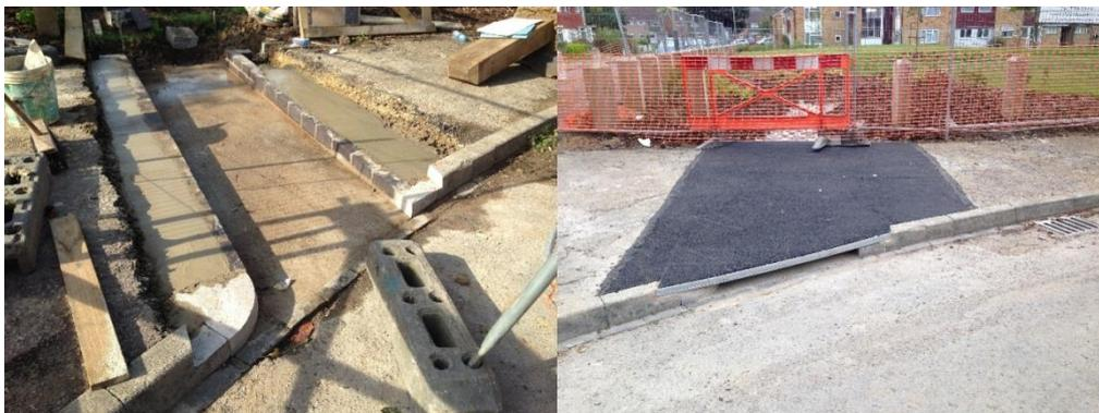
Fig 5: Inlet construction and complete with steel tray.
