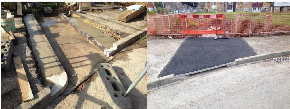
Fig 5: Inlet construction and complete with steel tray.
