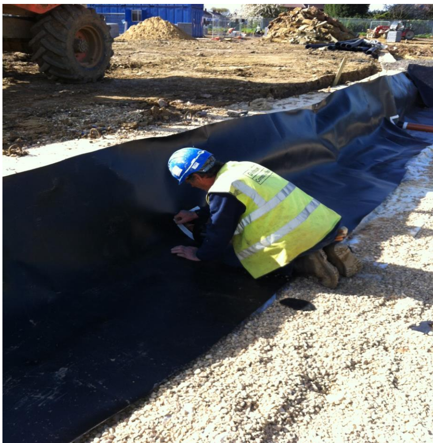
Fig 2: Taping up of private water inlets in impermeable liner
