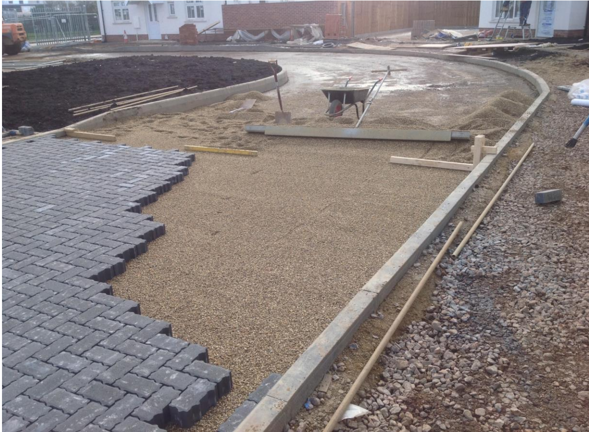
Fig 6: Laying the permeable blocks
