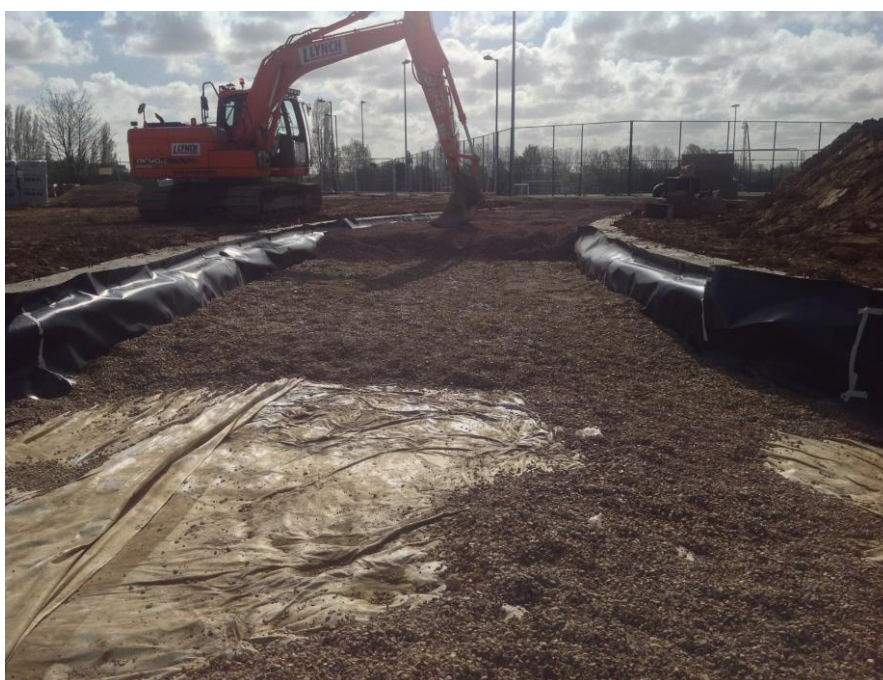
Fig 3: Laying of permeable sub-base
