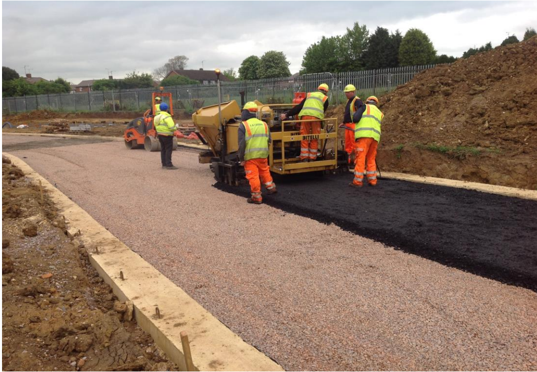
Fig 4: Laying of DBM on permeable sub-base
