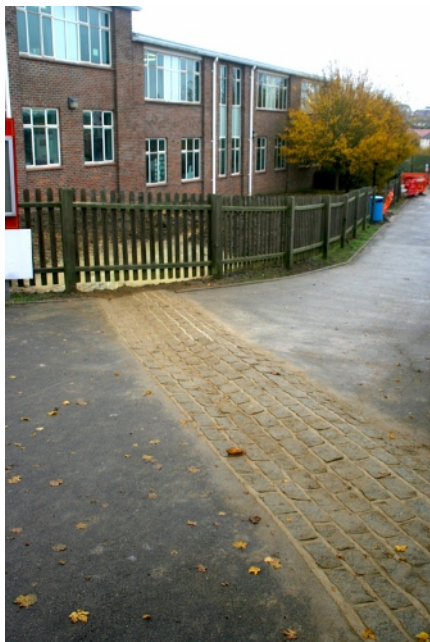
Figure 4: Granite sett flow diverter comprising combined channel and hump in a wave-like formation. The channel intercepts overland flow and diverts it to the raingarden basins beyond the fence (shown during construction).
