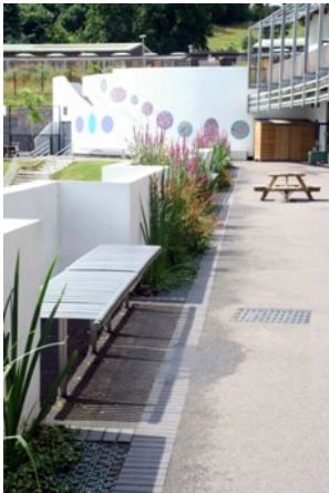
Figure 2 Permeable paving in school car park (Bob Bray)
