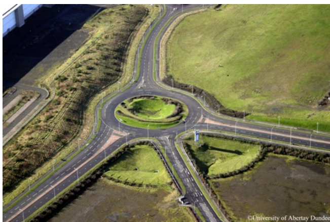
Figure 1 Detention basin DEX Roundabout (University of Abertay/SUDSNET)
