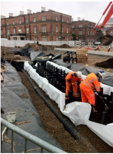
Figure 2: Construction of tree pit
