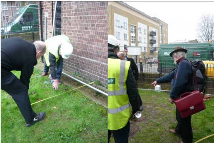
Figure 1 Marking out the layout of the rain garden
