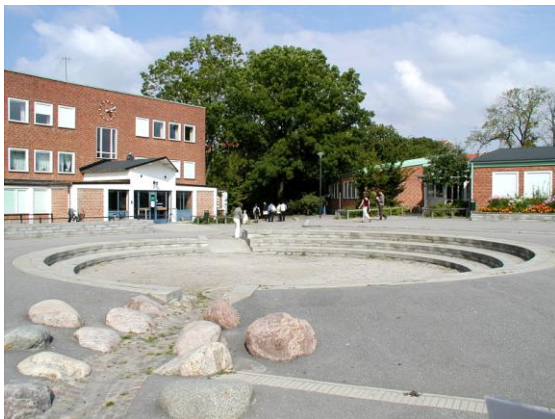
Figure 6 An auditorium in a Swedish school playground that also acts as a detention basin during heavy rains (courtesy Dick Fenner)
