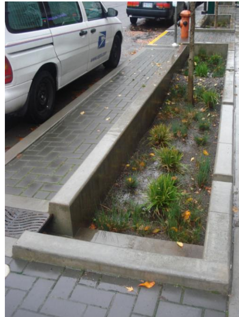
Figure 4 A recently constructed stormwater planter taking highway and footpath surface water on a street in Portland, Oregon
