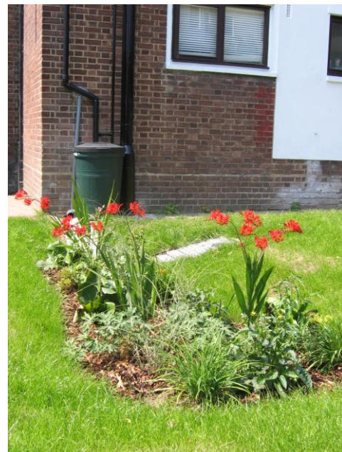
Figure 5 Rain garden built in Ashby Grove, London to collect roof water and infiltrate into the ground
