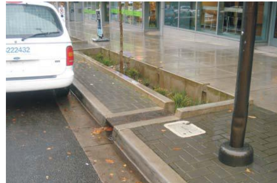
Figure 3 A recently constructed stormwater planter on a street in Portland, Oregon
