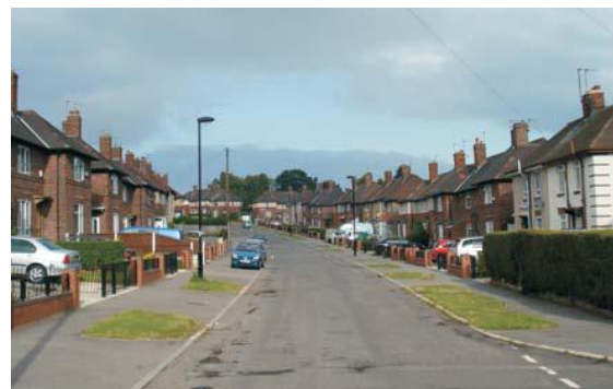
Figure 1 A typical UK suburban street where recent resurfacing works have taken place and a missed opportunity to manage the surface water
