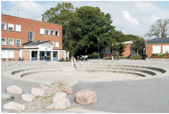
Figure 4 An auditorium in a Swedish school playground that also acts as a detention basin during heavy rains (courtesy Dick Fenner)
