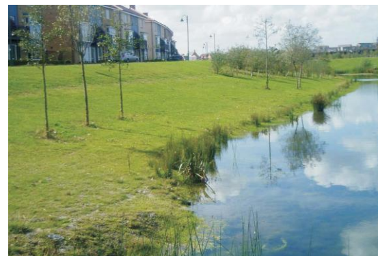
Figure 9 A SuDS pond with a shallow gradient
