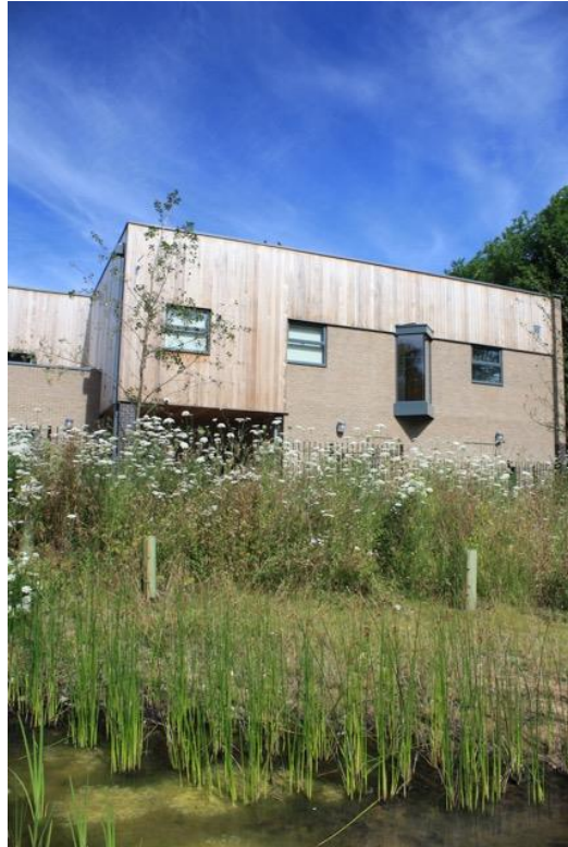
Figure 10 The Swales continuing to work well
