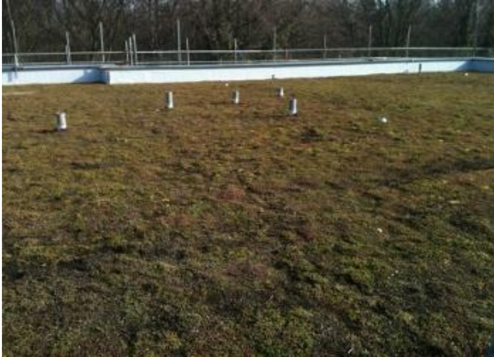
Figure 3 Biodiversity green roof. An all in one modular green roof system with an extensive sedum and lightweight soil-less wildflower mat laid over a 79-80mm substrate
