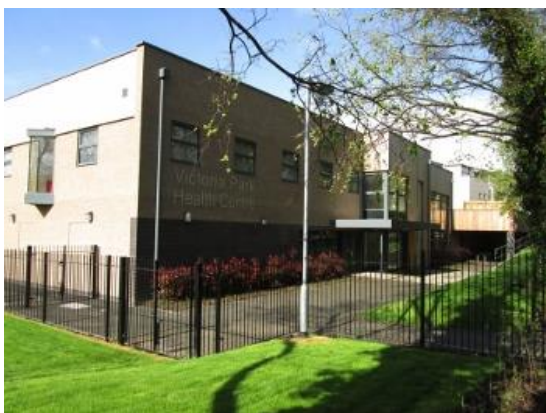
Figure 1 Victoria Park Health Centre main entrance
