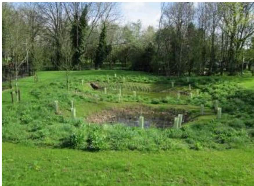
Figure 7 The infiltration basin with wildflower turf and grass seeding
