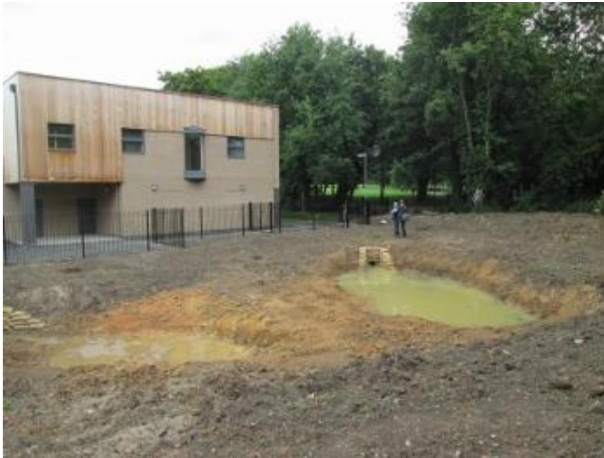
Figure 6 The infiltration basin during construction
