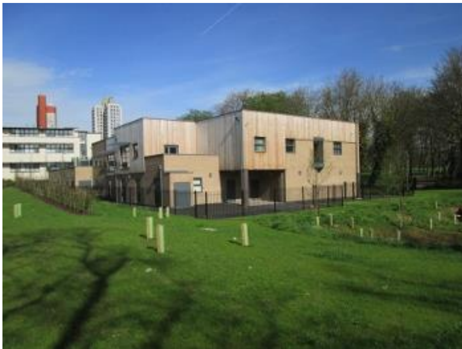
Figure 8 View of the health centre from the bund that partly screens it from the road
