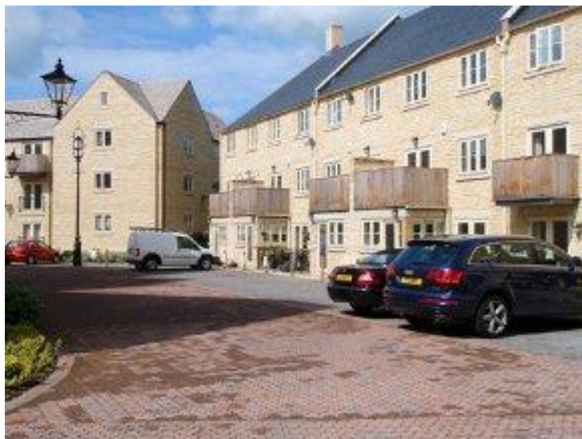
Figure 2 Car park using permeable paving (Bob Bray)
