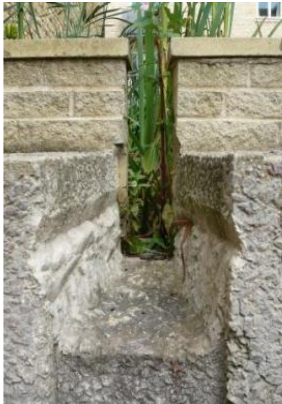
Figure 5 Outlet from rill to the River Welland
