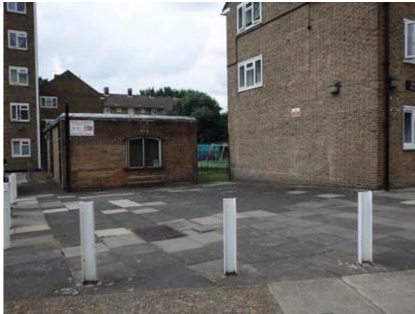
Figure 1 Prior to SuDS construction
