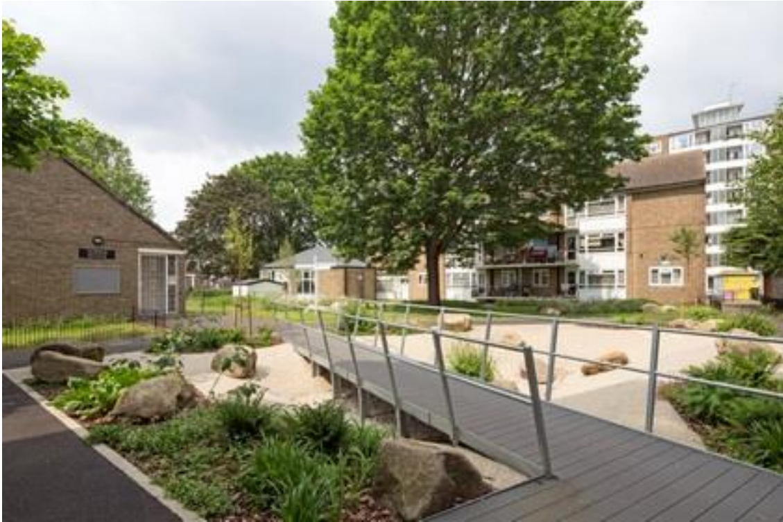
Figure 6 Stony detention basin
