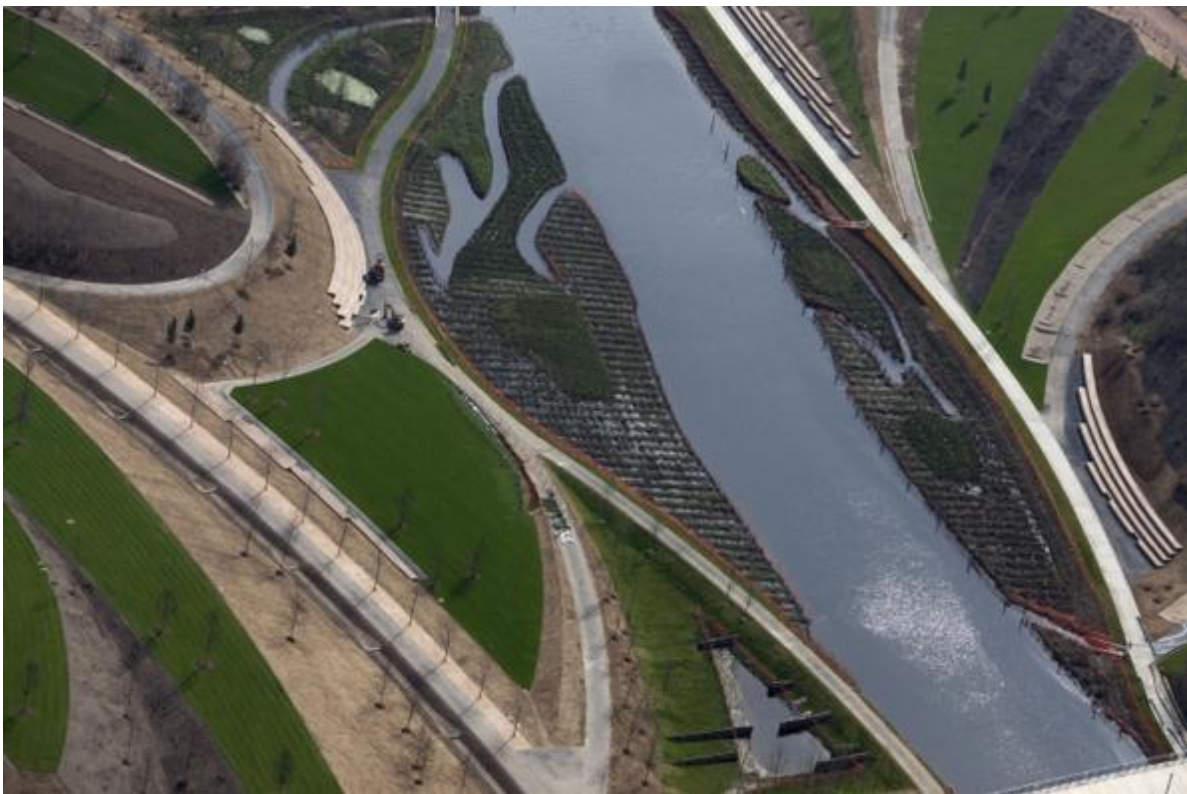
Figure 6 Overhead photograph of wetlands during construction (Barry Plowright)
