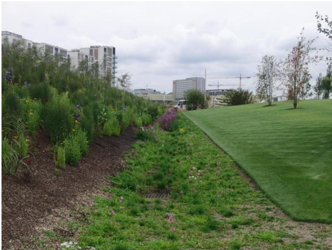
Figure 7 Photograph along planted swale (Barry Plowright)
