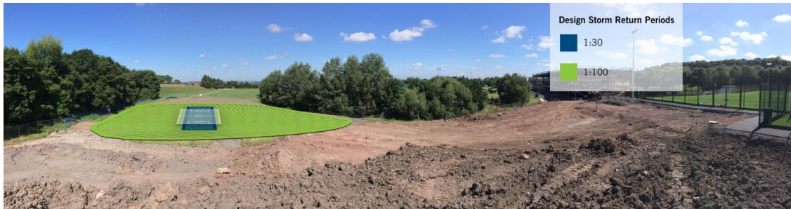
Figure 2 Looking out toward the proposed attenuation area
