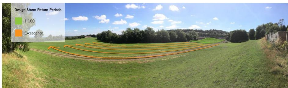
Figure 7 Greater than 1:100 plus climate change exceedance route and storage
