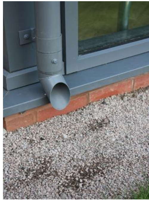
Figure 6 Disconnected downpipe (David Singleton)
