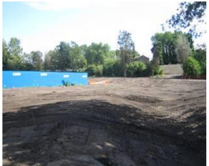
Figure 13 The main detention basin is downstream of this, which shows the care taken to grade swale sides (David Singleton)
