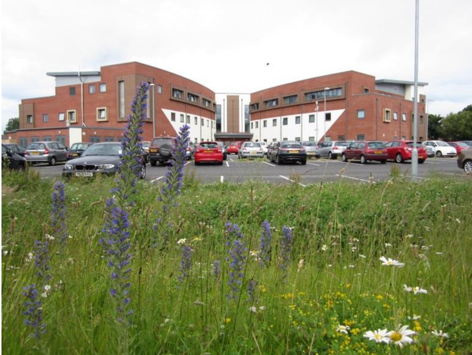
Figure 4 The innovative SuDS design takes advantage of the nature of the site and the ecological quality has significantly improved
