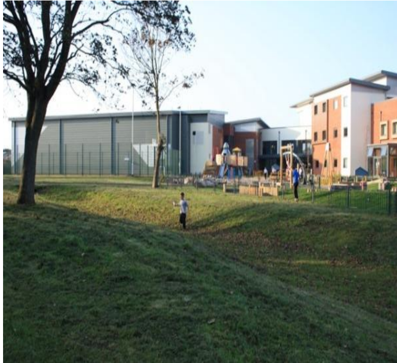
Figure 10 Low-flow swale (David Singleton)
