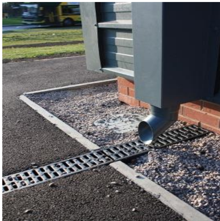
Figure 11 Disconnected downpipe to the sports hall channel (David Singleton)
