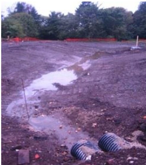
Figure 12 SuDS under construction (David Singleton)
