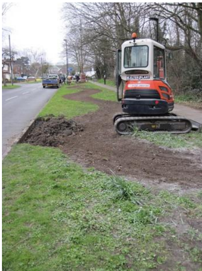
Figure 1 Constructing the swales
