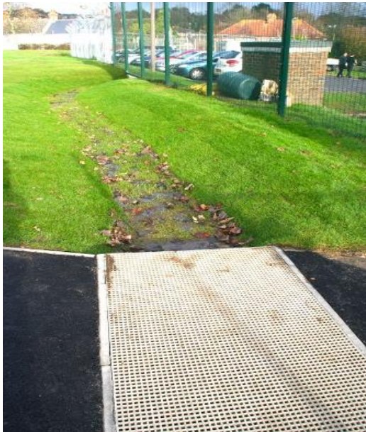
Figure 1 Bridge construction (before swale planting) allows shallow swale depth and grating surface intercepts path runoff
