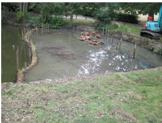
Figure 1 Reedbed construction
