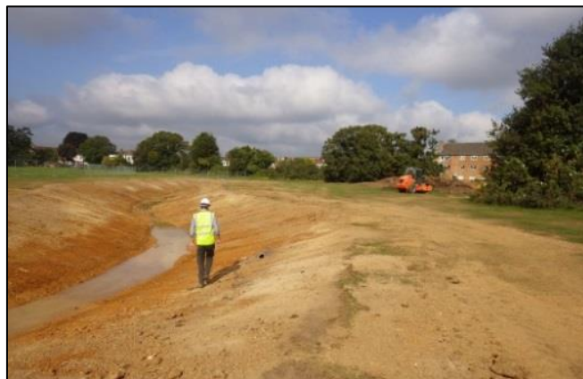
Figure 2 Firs Farm Site after completion of Phase 1
