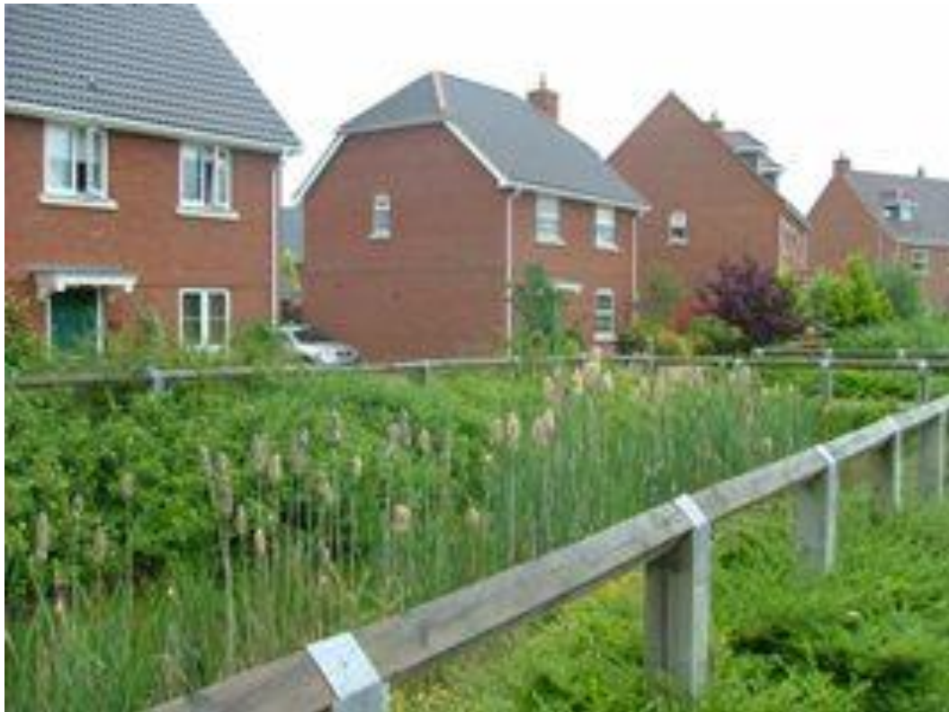
Figure 4 Swales run through the site providing drainage
