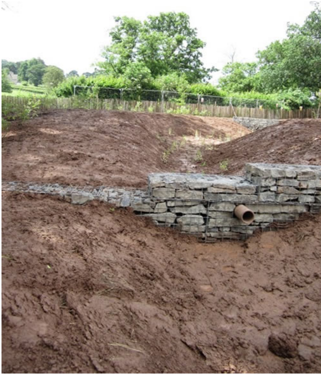
Figure 6: The treatment train of open swales and wetlands, separated by gabion baskets, filtering and infiltrating the water before discharging into the brook (During construction).
