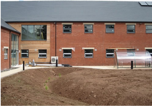
Figure 7: The swales were graded to be very shallow to enable mowing (During construction).
