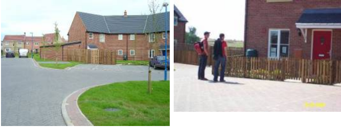
Figure 1 Permeable paving (Royal Haskoning)
