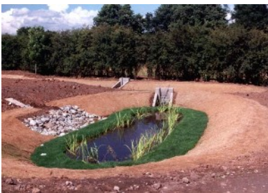
Figure 1 Spillage basin newly constructed (Bob Bray)
