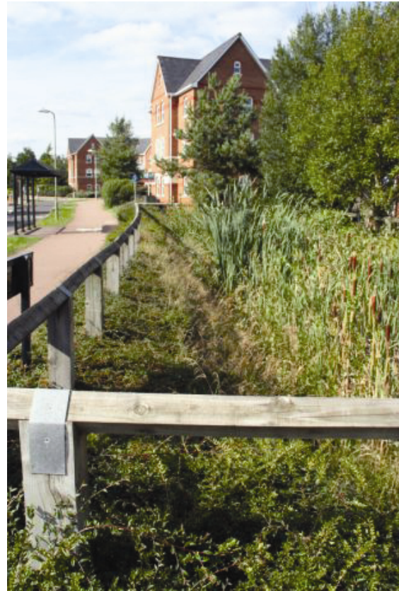
Figure 2 Elvatham swale (courtesy Bob Bray, Bob Bray Associates)
