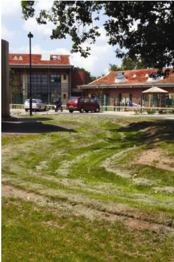
Figure 1 Birchen swale with view of the green roof (courtesy Bob Bray, Bob Bray Associates)
