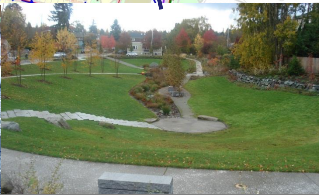
Detention basin in open space
