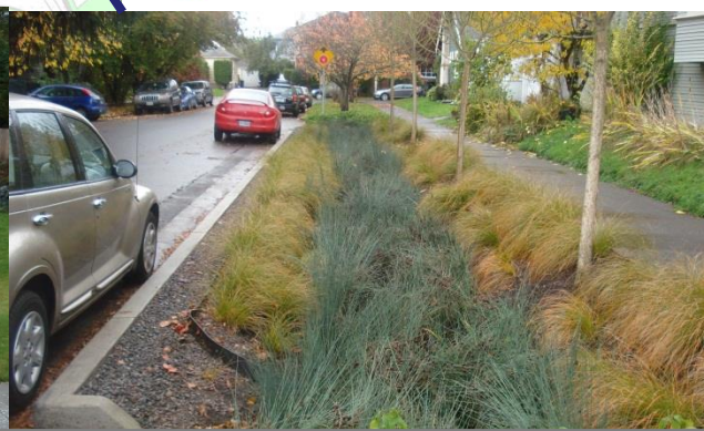
Bio-filtration swale along highway
