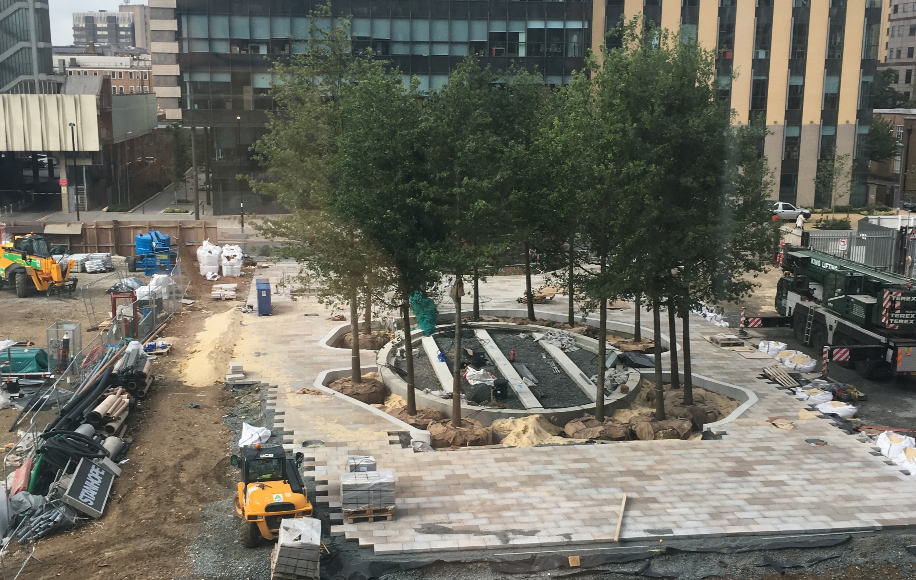
SEPTEMBER 2016 | SOFT LANDSCAPE INSTALLATION
