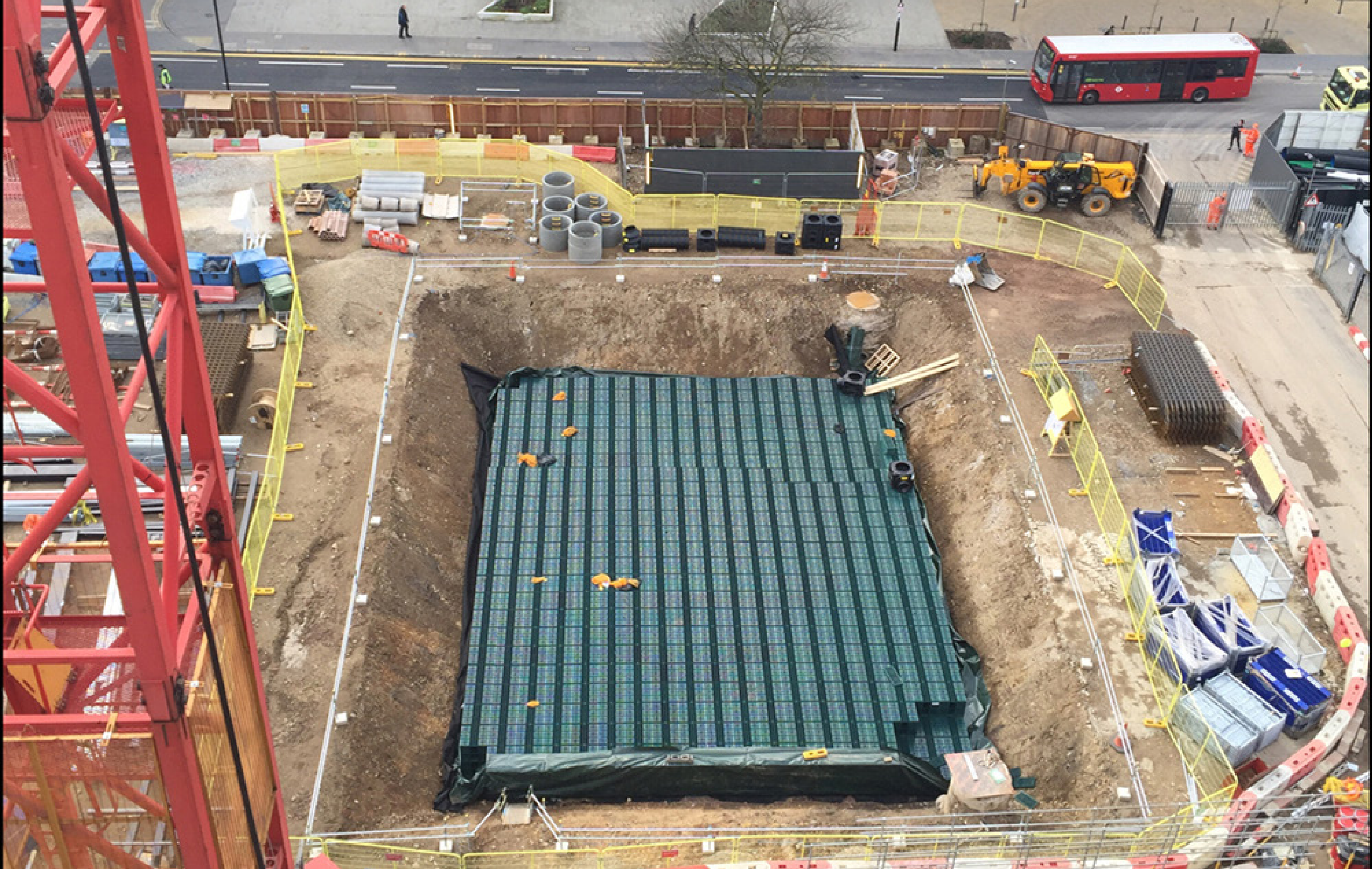
MARCH 2016 | ATTENUATION CRATE INSTALLATION
