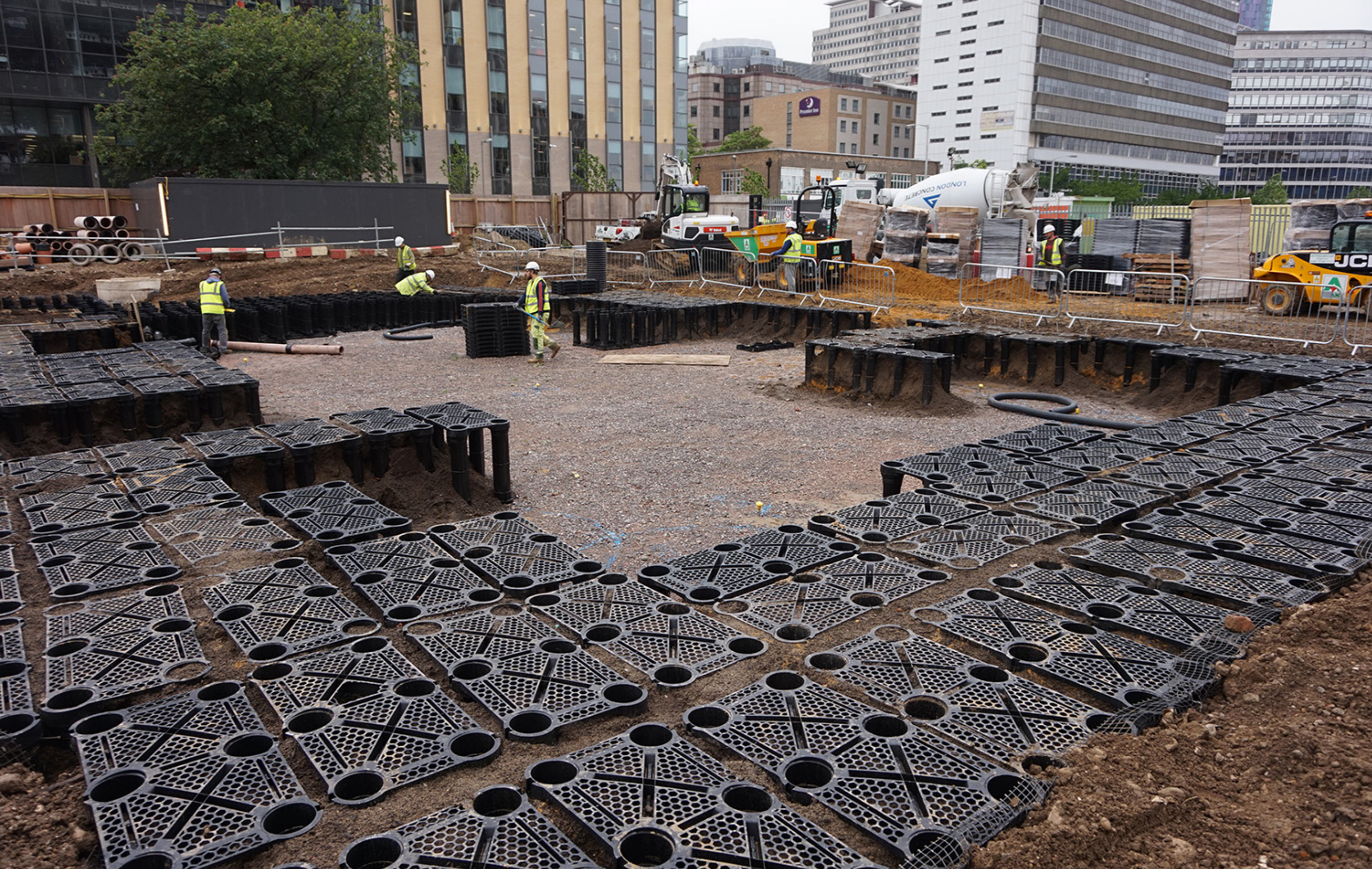
JUNE 2016 | SOIL CELL INSTALLATION
