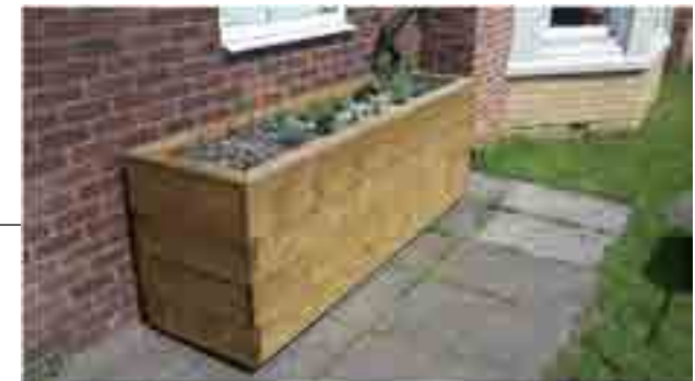
Northwich Youth Centre SUDS planter, with soakaway
