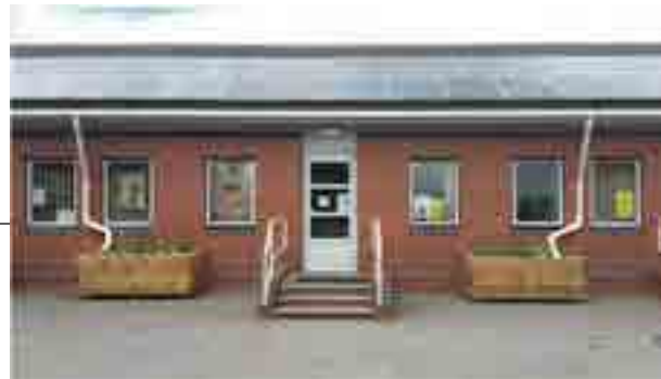
Charles Darwin Community Primary School SUDS planters
