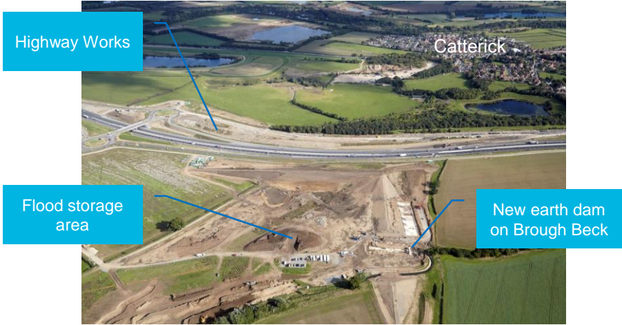
Highways England partnership funding of Environment Agency Scheme
