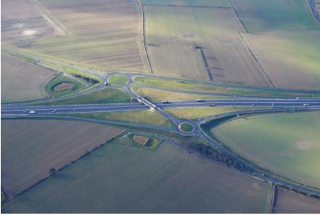
Baldersby East and West Ponds visible highlighting forebay with reeds and secondary dry retention storage area,
