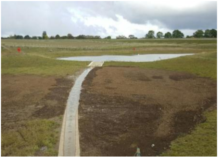
Angleham pond overflow
