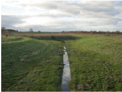
Base of detention basin
