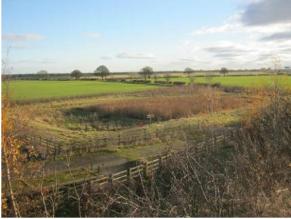
Attenuation pond with reed planted forebay
