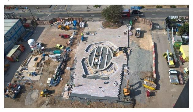
Fig 4 Grit-jointed permeable paving installation, September 2016. © Lendlease
