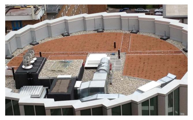
Fig. 8: Mixed finish roof
