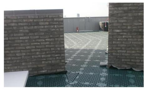
Fig. 3: Installed Void formers fitted in tight working environments
