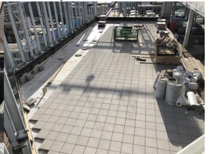
Level 50 terrace area with paved finish
