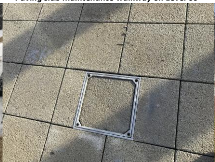
Level 50 chamber lid recessed into paving
