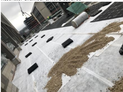
Installing water flow reducing layer to Level 50
