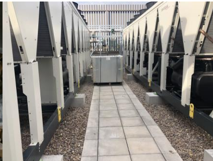
Paving slab maintenance walkway on Level 60
