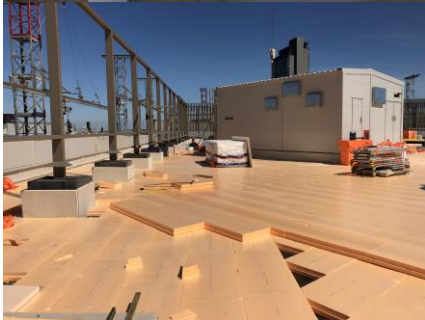
Insulation boards installation Level 60
